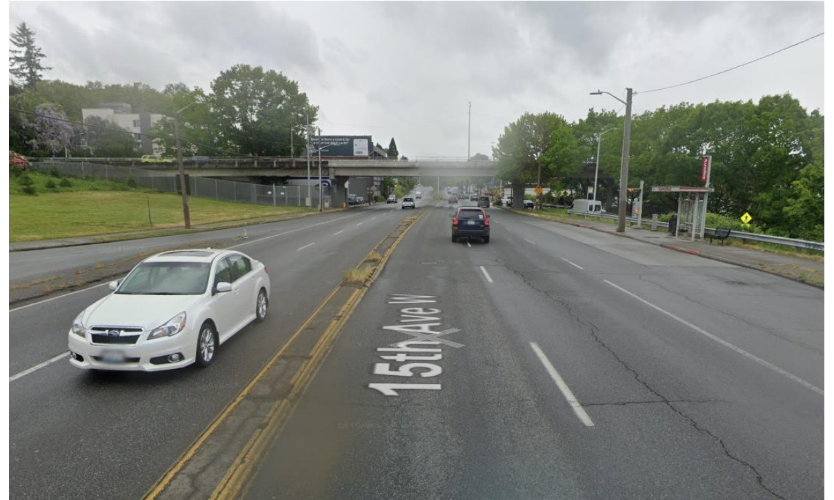
15 th Avenue W south of Ballard Bridge
